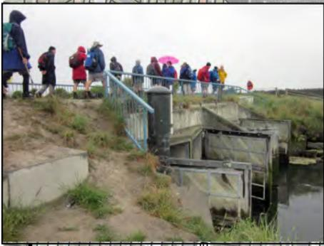
Foreshore barrier elevation should be around 1.5 m AHD, which corresponds to the 1% AEP Brisbane Water Flood Level
