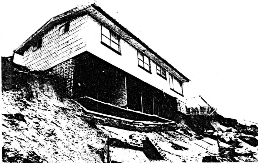
**Figure 10: House severely damaged by dune erosion at Wamberal-Terrigal Beach in 1974
