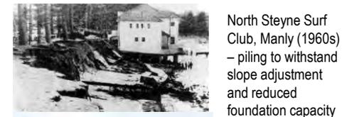
North Steyne Surf Club, Manly (1960s) – piling to withstand slope adjustment and reduced foundation capacity
