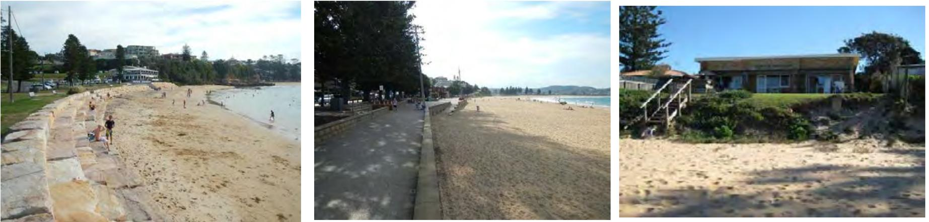
**Figure 1:** Stepped sandstone block seawall along the southern section of Terrigal Beach (left) and block seawall and promenade along the central section of Terrigal Beach (right)
