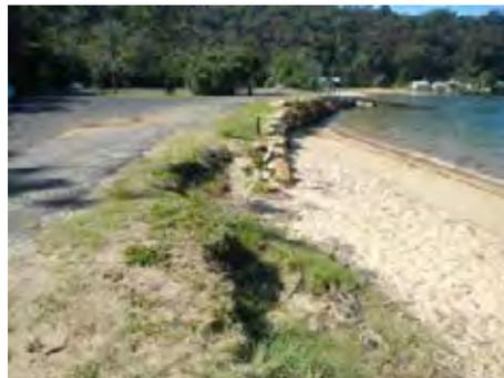
7. Existing erosion protection works at boat ramp and minor erosion adjacent to works
