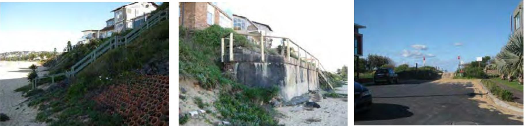
**Figure 2:** Rock gabion and terracotta pipes (left) and concrete retaining walls (right) constructed in front of properties
