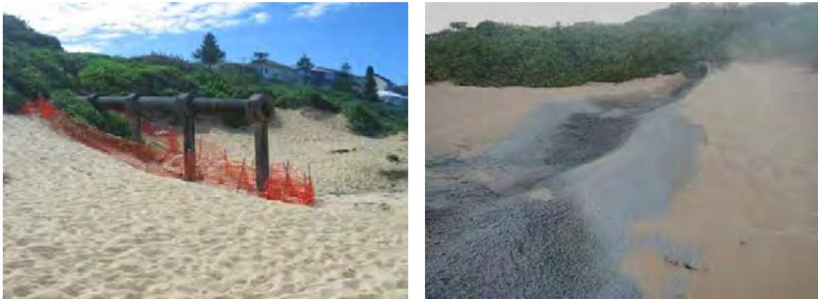
**Figure 2:** Piled stormwater outlet (left) replaced with a stormwater outlet within the dune system and a concrete apron in front of a stormwater outlet (right)
