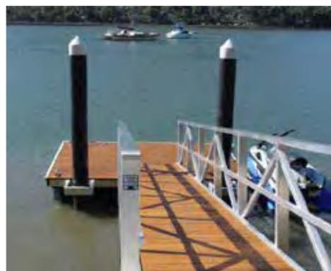
Floating timber pontoon example
