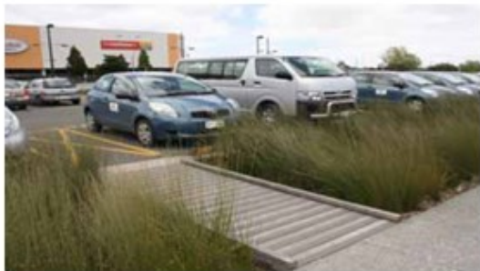
Raingardens in car-park, New Zealand
