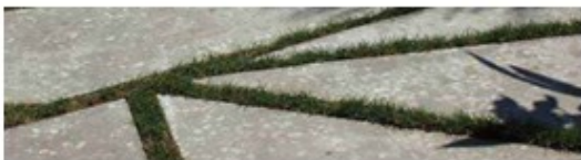
Large gaps between pavers can treat runoff at the source
