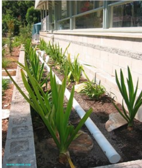
Planter box bio-retention system, Sydney
