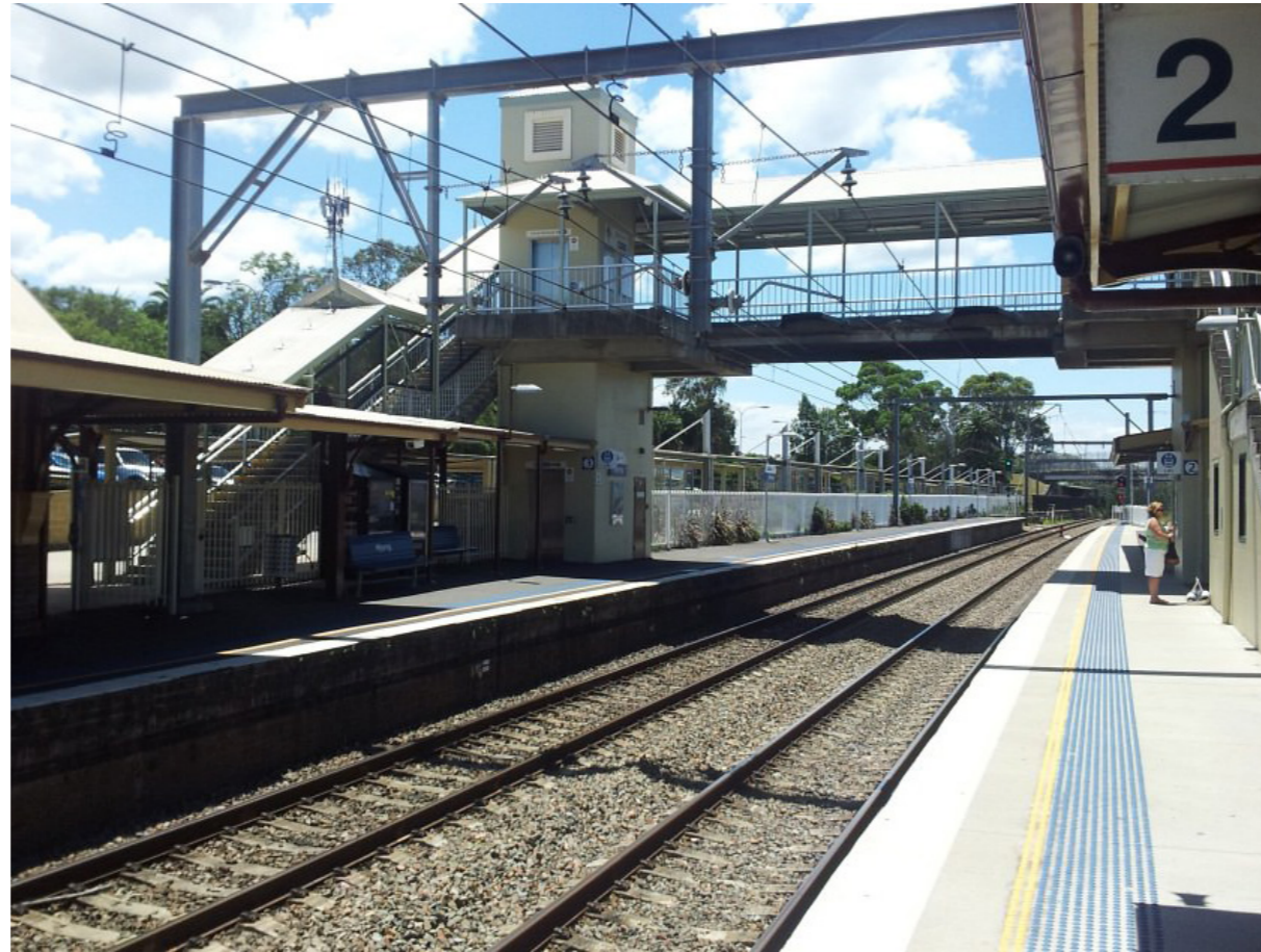
Wyong train station
