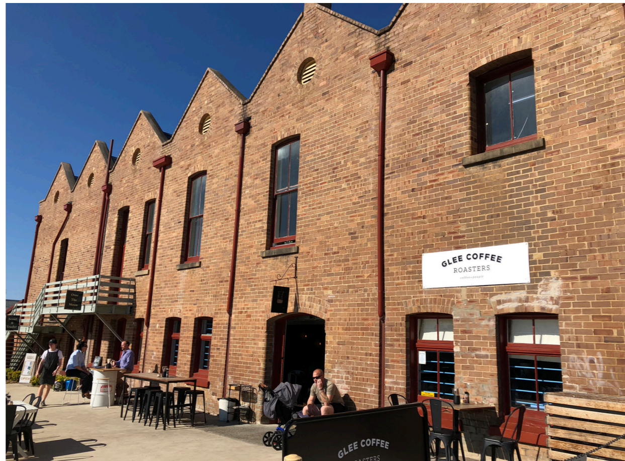
Chapman building, Wyong
