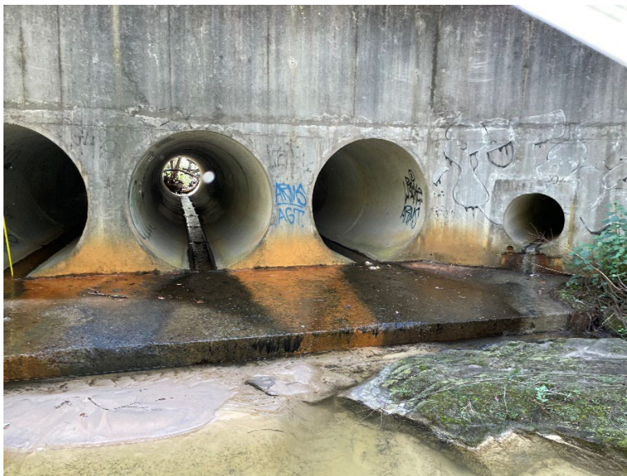
Figure 2-12: Cross-Drainage Structure along Somersby Fall Road at Piles Creek
