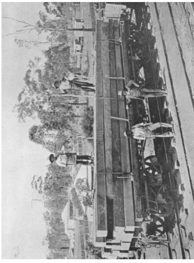
Figure 5.3 Square turpentine beams on railway wagon at Wyong Railway Station, c1909. Turpentine was used extensively in wharves and jetties on the Central Coast and in Sydney. Timber from Stinson's mill. (Source: Central Coast Memories, Central Coast Library Service)
