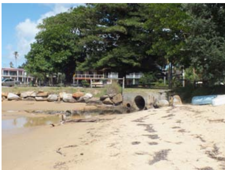
Figure 4.54 Concrete stormwater outlet near Beach Road.
