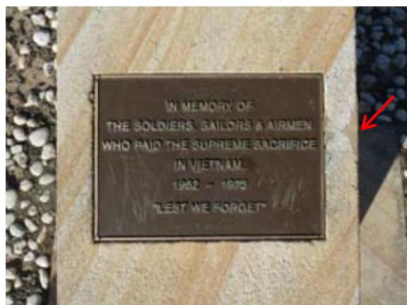
Figure 4.67 Bronze plaque on upper, slope face of the memorial. A small epoxy patch repair can be seen on the stone to the right side of the plaque (red arrow).
