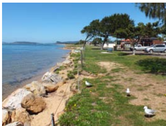
Figure 4.58 Straight sandstone revetment at the north end of the precinct; view from the north.
