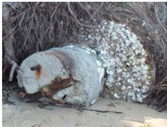
Figure 4.43 Concrete block bolted to the west end of the vessel, which is covered with oyster shells.
