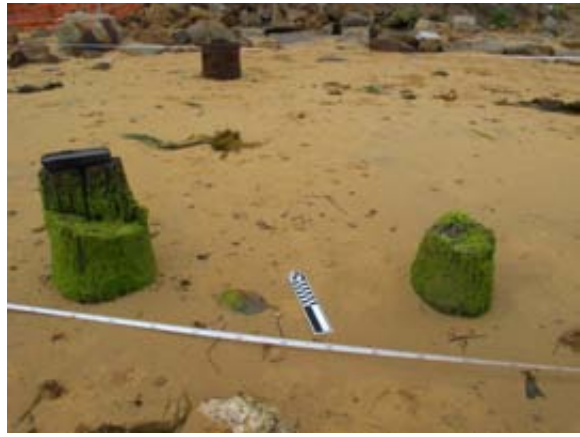
Figure 4.33 Series of paired timber piles, with one to the left showing a rebate for cross bracing; view from the south. (Source: ANMM 2012)
