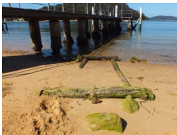
Figure 4.31 Slipway carriage or cart, partially buried in the sand; view from the northeast.
