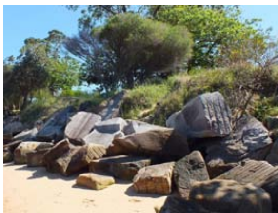
Figure 4.16 Retaining wall, with dumped sandstone quarry blocks along the eastern part of Lance Webb Reserve.
