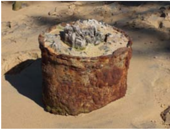
Figure 4.32 Timber pile with steel drum and concrete collar.
