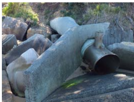
Figure 4.18 Damaged stormwater outlet, at the south end of Schnapper Road.
