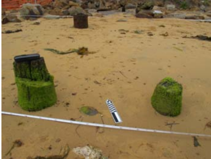
Paired timber piles in foreground of photograph, one to the left showing a rebate for cross bracing, Ettalong Beach, looking north
