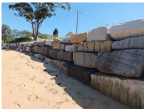
Figure 4.15 Retaining wall, built with large, castoff sandstone quarry blocks along the western part of Lance Webb Reserve.
