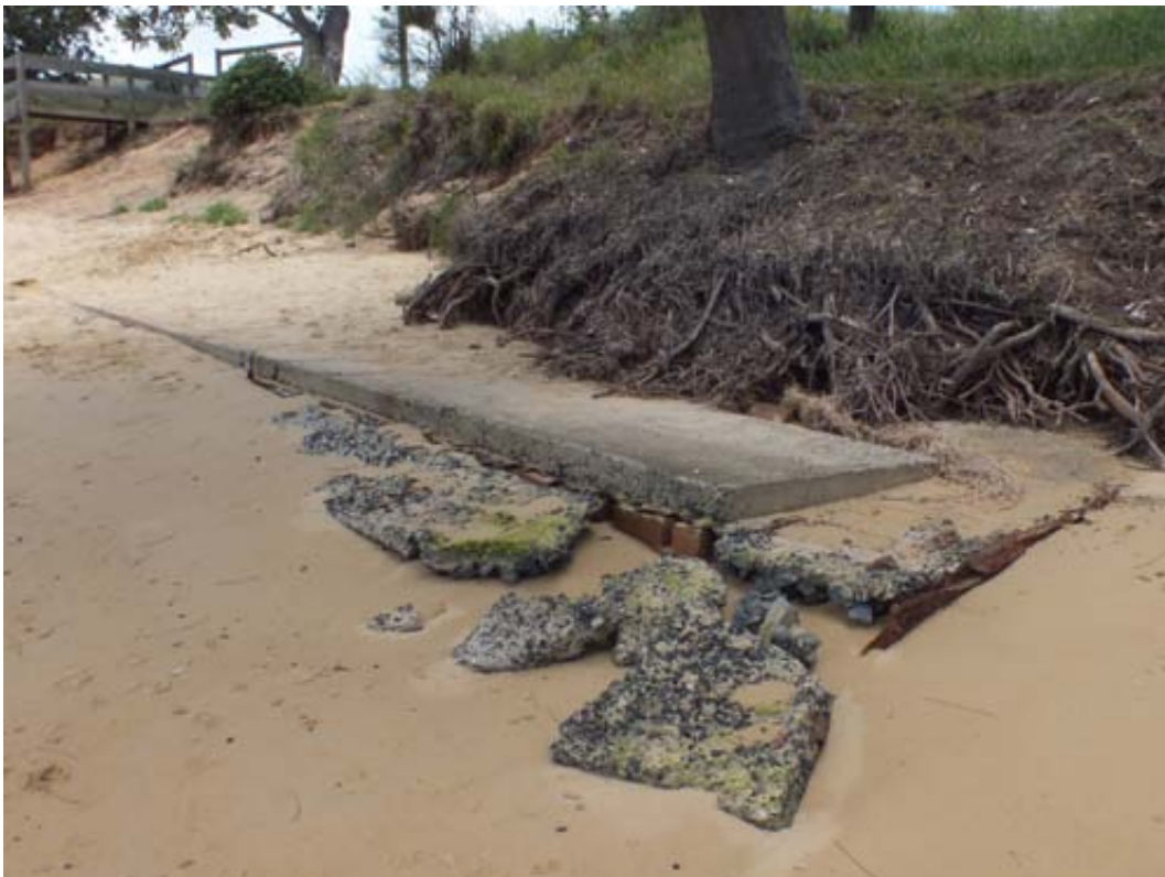
Figure 4.45 Brick footings have been exposed at the southeast corner of the slab. A sheet of corrugated metal is between the brick and the concrete.
