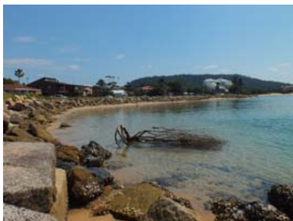
Figure 4.57 Curving sandstone revetment at the south end of the precinct; view from the south.
