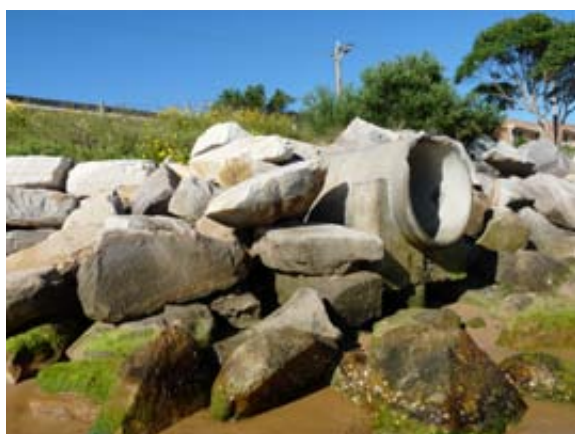
Figure 4.17 Concrete stormwater outlet pipe, at the junction of two sections of retaining wall.
