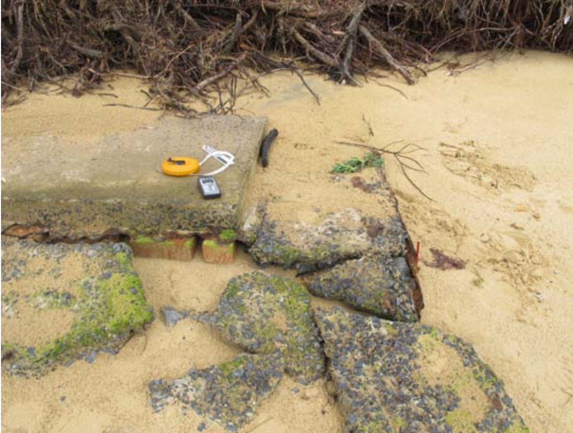
Feature Three looking north showing the brick footings
