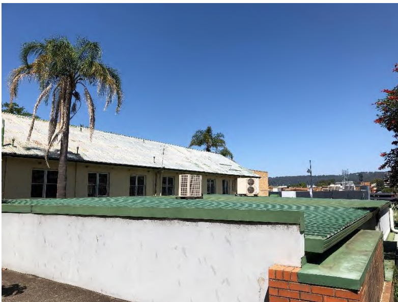
Photograph 2: Rear view of existing building looking west
