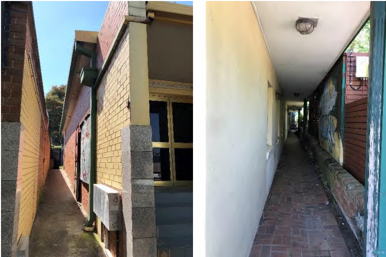
Photograph 7: Existing unrestricted access points to the existing building
