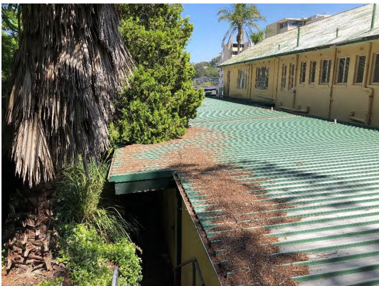
Photograph 6: Southern elevation of existing building and view of enclosed public pathway
