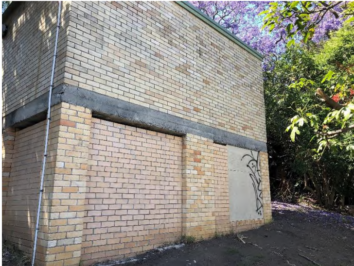
Photograph 3: Detached garage to be demolished
