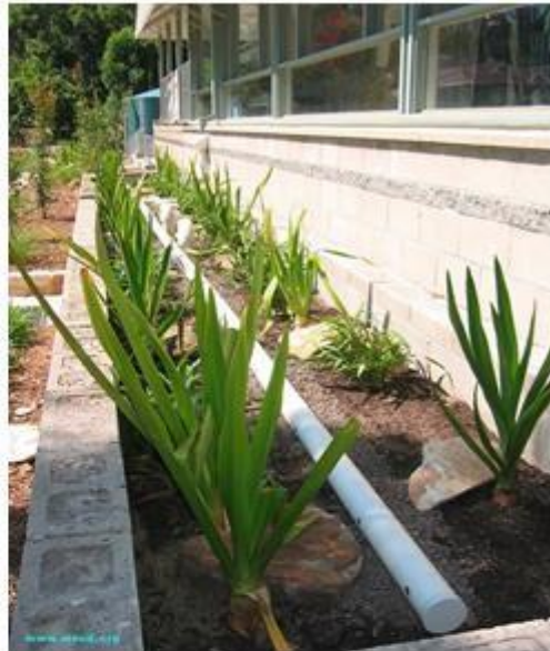
Planter box bio-retention system, Sydney
