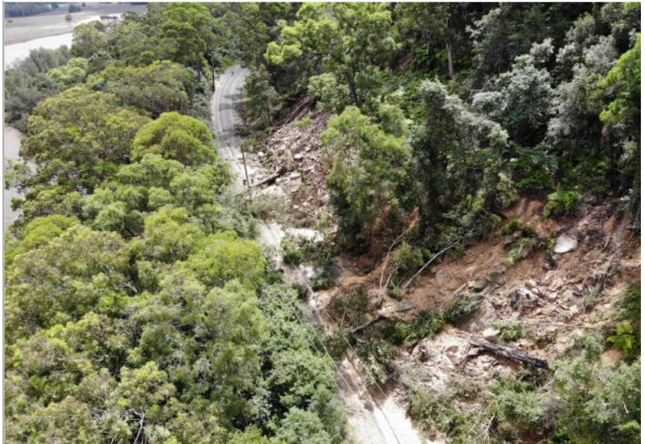
Figure 1-2 A view of the damaged slope from above prior to initial clean up
