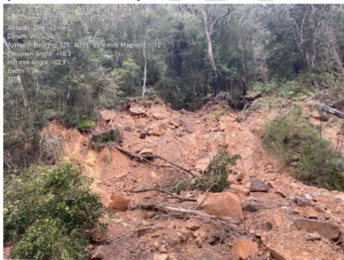
Figure 1-5 View looking upslope-Note buried cliff line in centre of image
