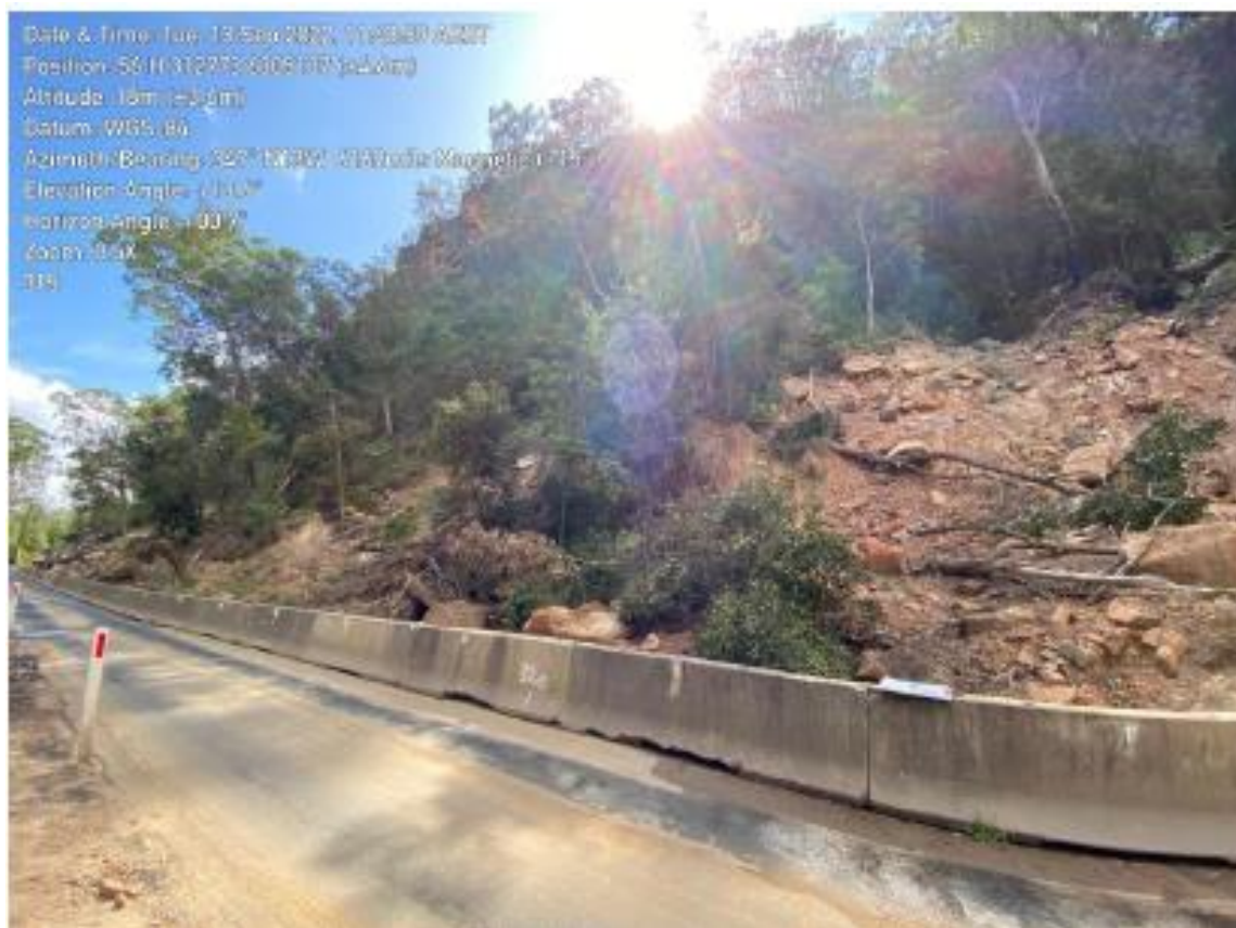
Figure 1-4 Views of the landslide looking north
