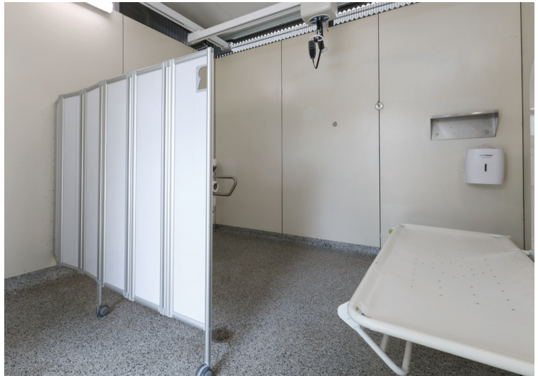
Image: An internal view of a Changing Place with privacy screen, adult changing table and hoist.
