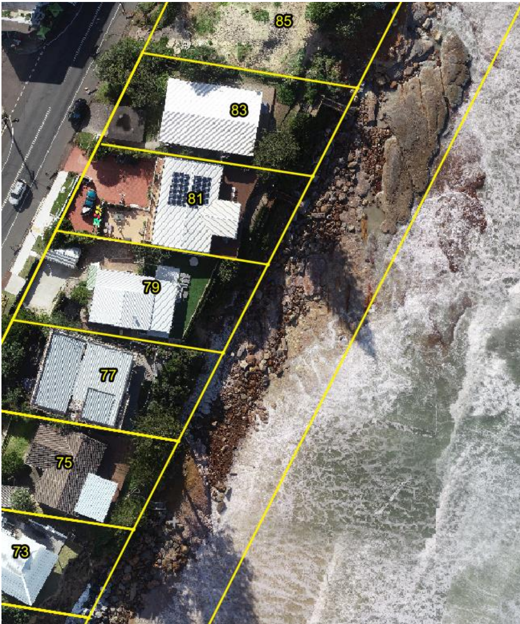
Figure B. 2: Claystone outcrop located between 73-87 Ocean View Dr. Imagery from 19 Jul 2020 Drone Survey.
