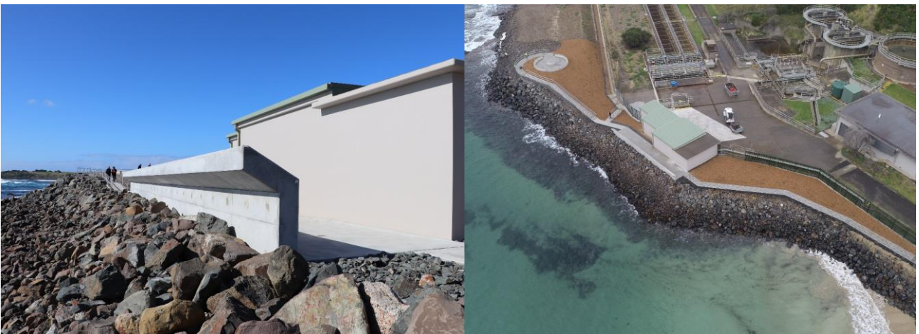
Figure 3.3: Port Kembla basalt rock revetment constructed 2020. Images provided by MHL and James Carley (WRL).
