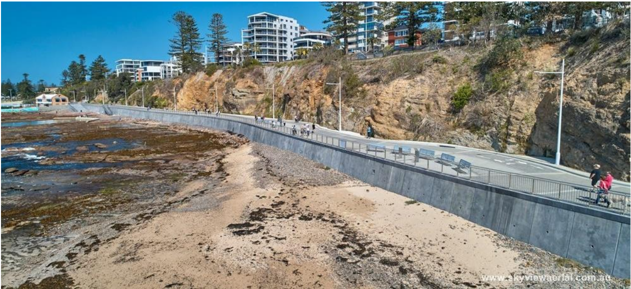
Source: www.skyviewaerial.com.au - https://www.wollongong.nsw.gov.au/council-projects/ongoing-projects/the-blue-mile Figure 3.12 Vertical wall with promenade at Blue Mile pathway, Wollongong. Completed 2018. Image provided by Wollongong City Council.
