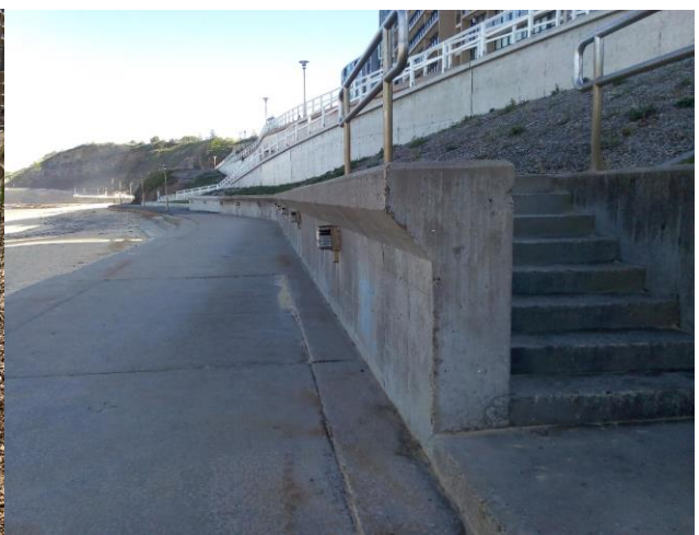
Figure 3.14: Tiered vertical wall (with stepped sections) and promenade at Newcastle Beach showing landward wall wave return on right. Images provided by Paul Donaldson (Central Coast Council) and MHL.
