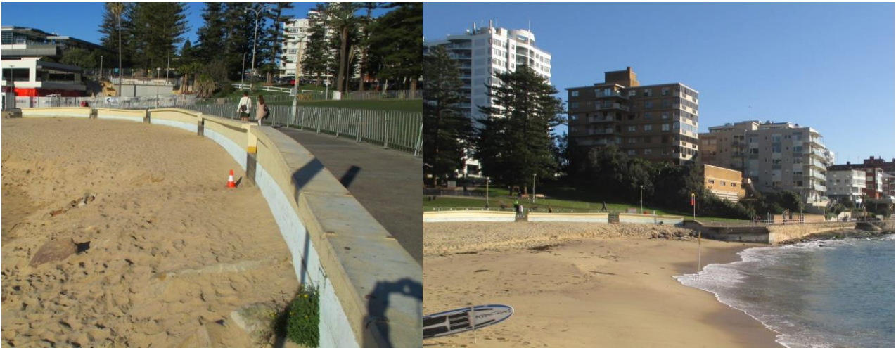
Figure 3.8: South Cronulla vertical seawall with wave return. Images provided by MHL.
