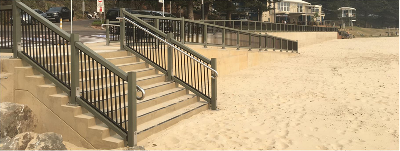
Figure 3.7: Flynn's Beach, Port Macquarie vertical seawall design with ramp and stepped access. Constructed 2019. Images provided by Port Macquarie-Hastings City Council.
