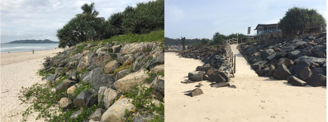
Figure 3.2: Rock Revetments at Belongil Byron Bay (left) and Lennox Head (right). Images provided by James Carley (WRL).
