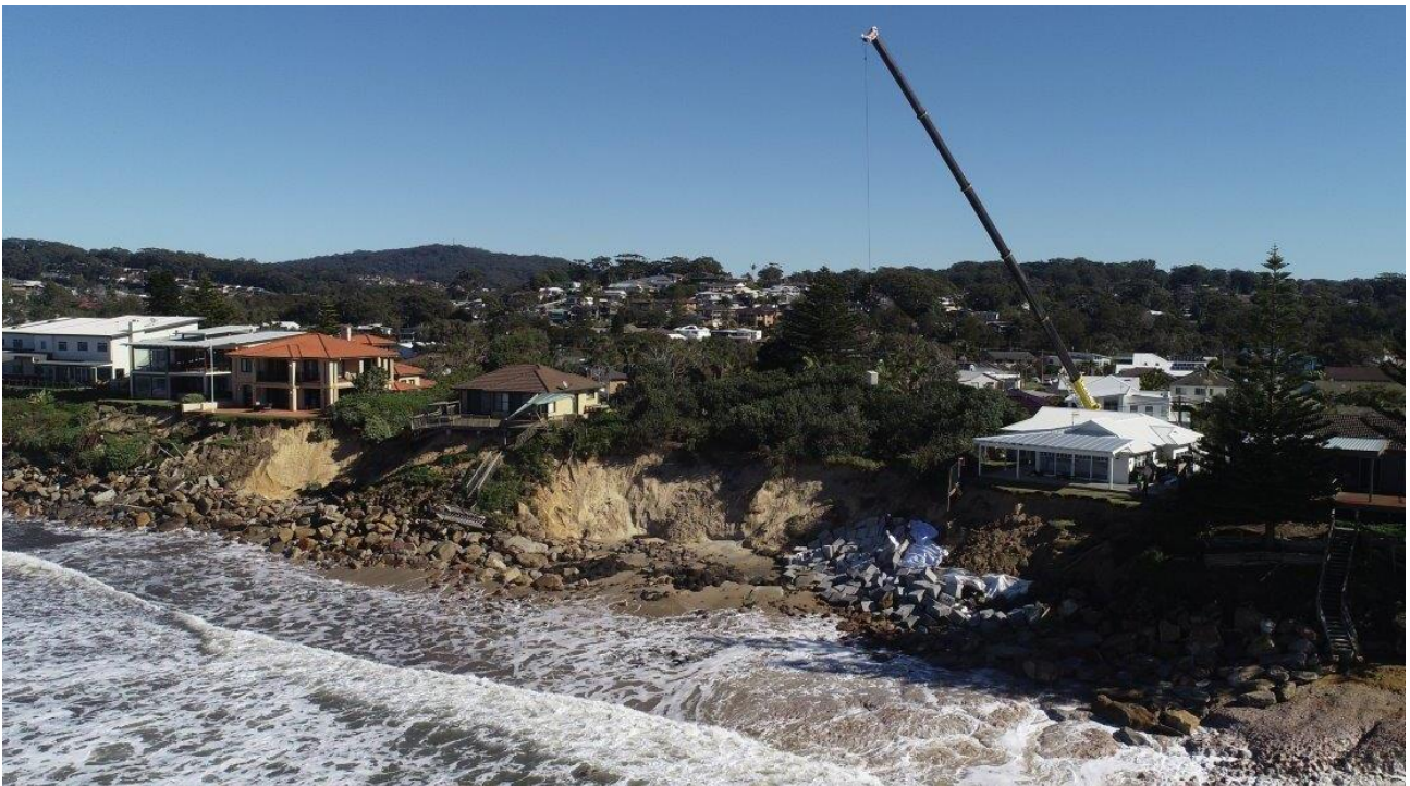
Figure 5.8: Wamberal Beach after storm erosion on 20 th July 2020. MHL drone survey.
