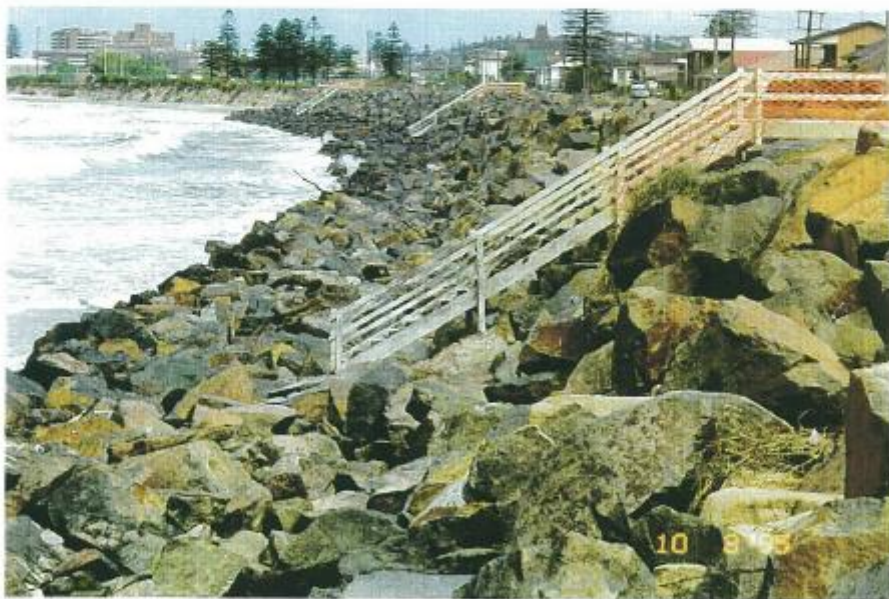
b) Typical Post-Storm Conditions
