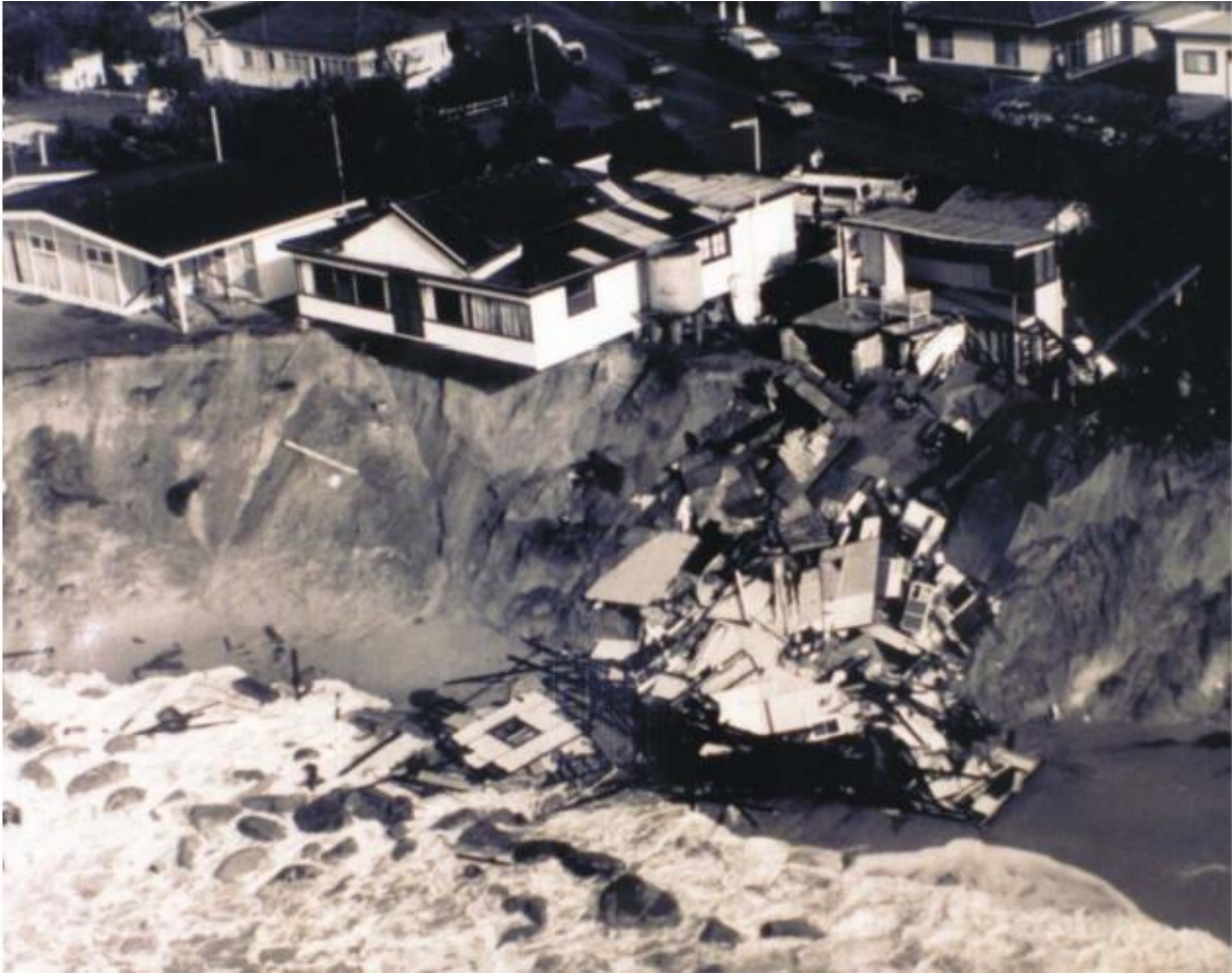
Figure 3.2 Collapse of house at 23b Ocean View Drive Wamberal in June 1978 (News Limited)
