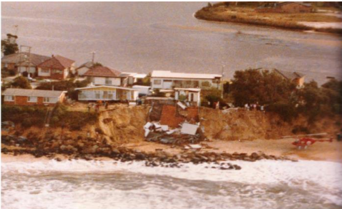
Figure 3.3 Collapse of house at 23a Ocean View Drive Wamberal in June 1978
