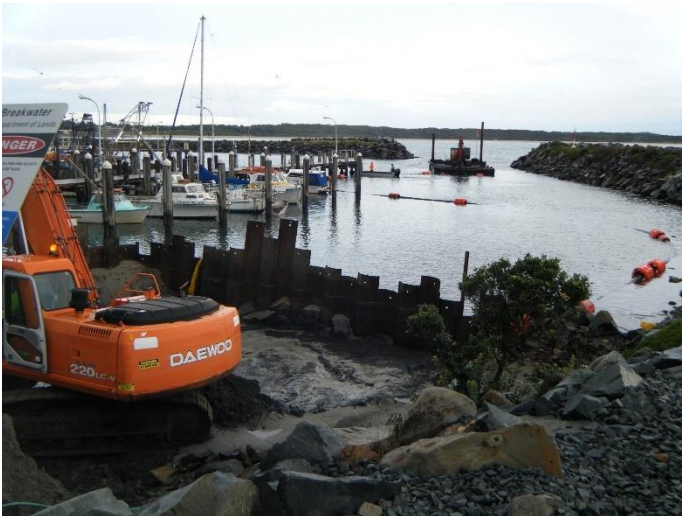
Photo 2 Excavator and barge arrangement
